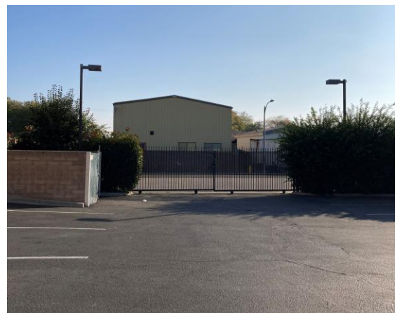
Gate access to Houston Lane
