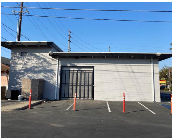
Facing rear of building
